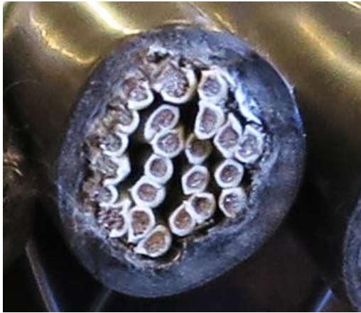
Photo 2. Prior to test, cross section.
